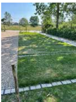
Camping de Savonnières – Parking - Travaux 2022
